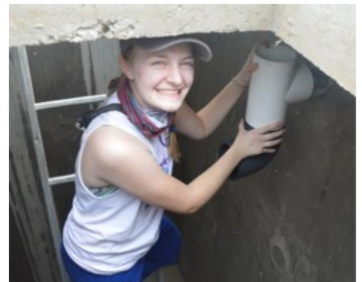
with Glenn. Power lines were strung from the solar panels to the work site. With help from Hope and Jase, I went down into the large tank (approximately 5x8x9 ft) along with Glen and McKenzie (at different times, cause come one, it’s a big tank but not that big) to install the piping that ensures even distribution of wastewater in the tank. Concrete was also poured at the old site.
